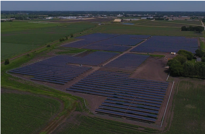
Southern Minnesota Municipal Power Agency's 5 MW Lemond Solar Station Owatonna, MN
